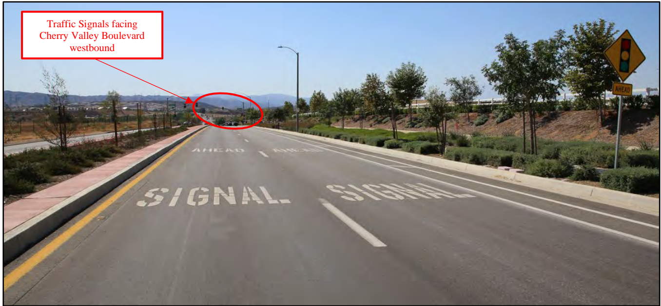
Figure 11. View of traffic signals facing Cherry Valley Boulevard westbound, 675 feet east of the signal lights.
